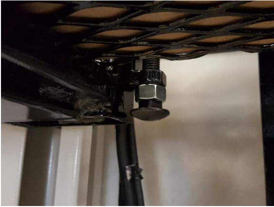
Figure 3, 4 5/8” carriage bolt – mechanical stop
