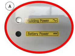
**on,** as the standard operating mode is to run on battery power. If the building power light is on, check that the batteries and inverter are functioning.
