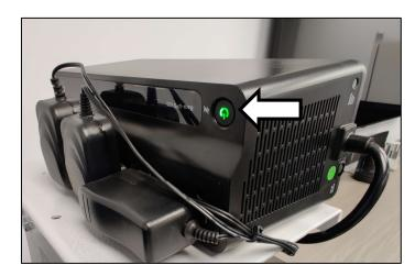
This UPS powers the emergency lighting, emergency alarm, and interlocks, **but does not power the lift**. In the envent of a loss of power, the lift will still need to be manually cranked to the nearest landing.
